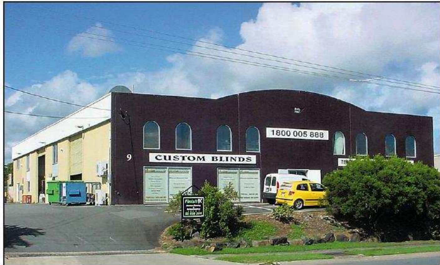
The three-unit Burleigh Heads industrial complex where Scafflink will relocate to the rear unit
