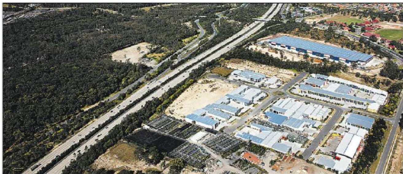
Supply running out . . . an aerial view of Coomera Business Park
